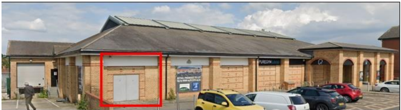
Figure 8 Existing Building [former Aldi prior to former Poundland] application unit shown in red square
