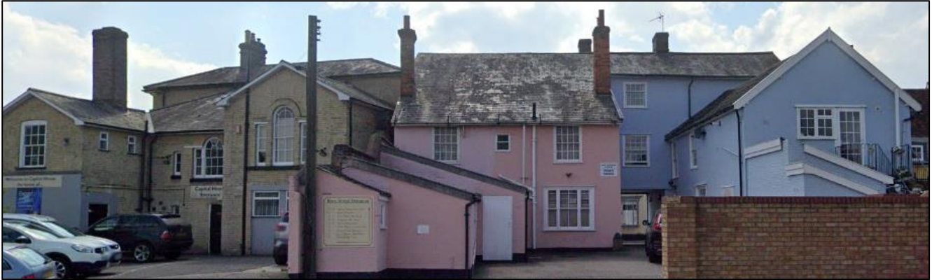
Figure 9 Rear of existing buildings in Bury Street
